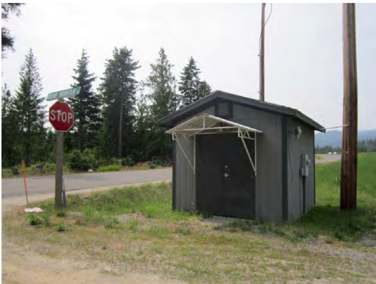
Photograph 99: Highland Flats booster station building
