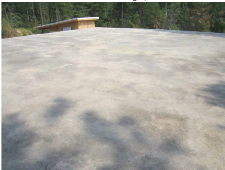
Photograph 81: Naples tank roof
