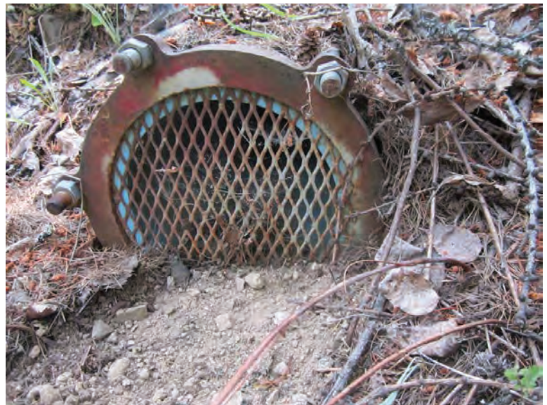
Photograph 68: Black Mountain reservoir screened drain
