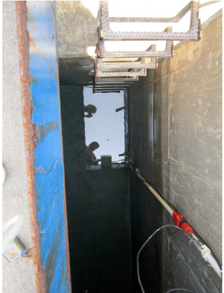
Photograph 50: Black Mountain reservoir interior
