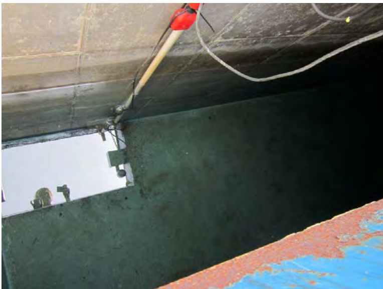
Photograph 51: Black Mountain reservoir interior
