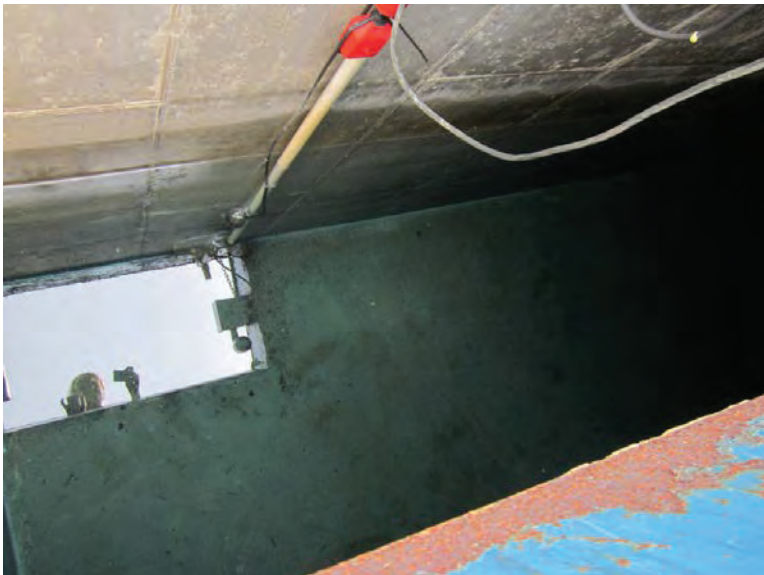
Photograph 51: Black Mountain reservoir interior
