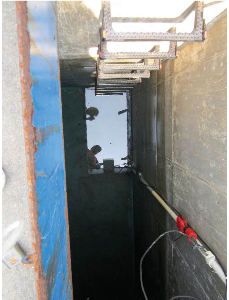
Photograph 50: Black Mountain reservoir interior
