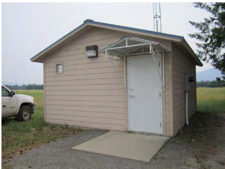
Photograph 47: Four Corners booster station
