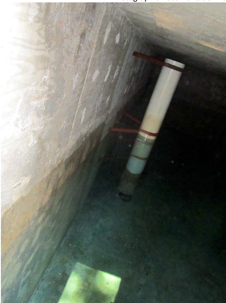
Photograph 85: Naples tank overflow
