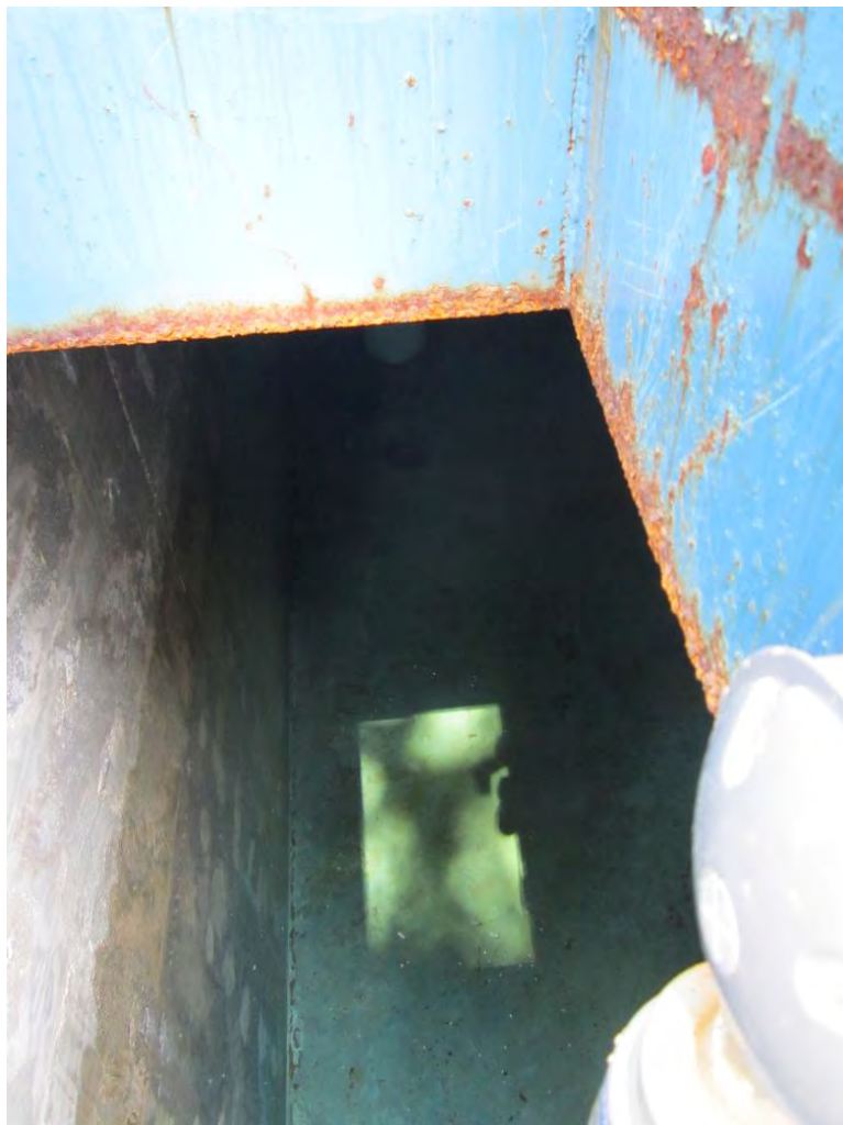
Photograph 82: Naples tank interior
