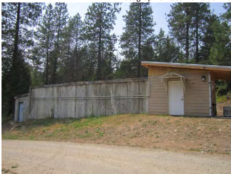
Photograph 73: Naples tank and booster station
