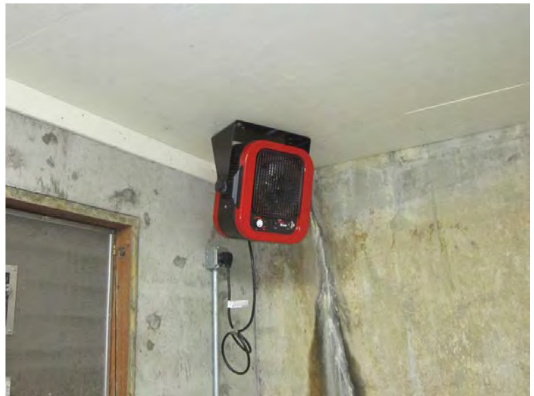
Photograph 64: Black Mountain booster station, thermostatically controlled heater
