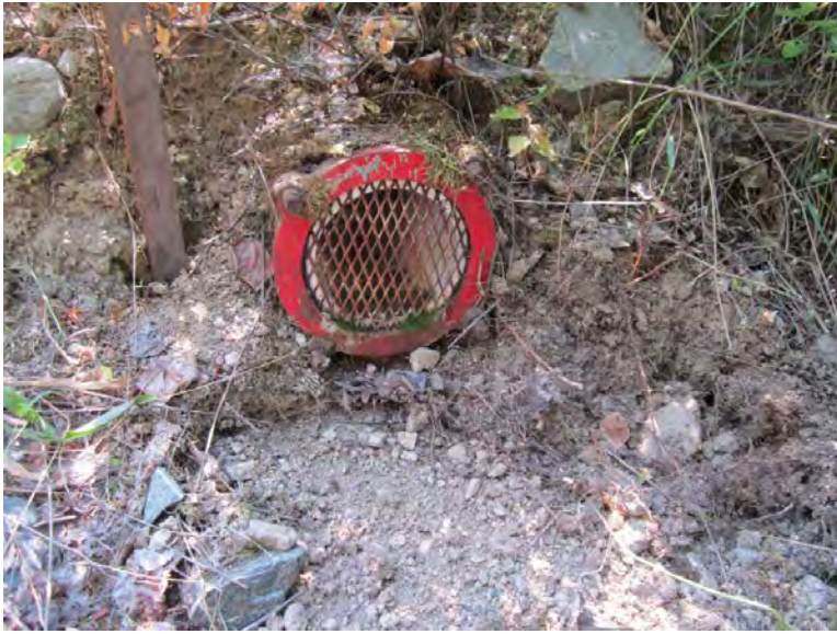
Photograph 69: Black Mountain reservoir screened overflow
