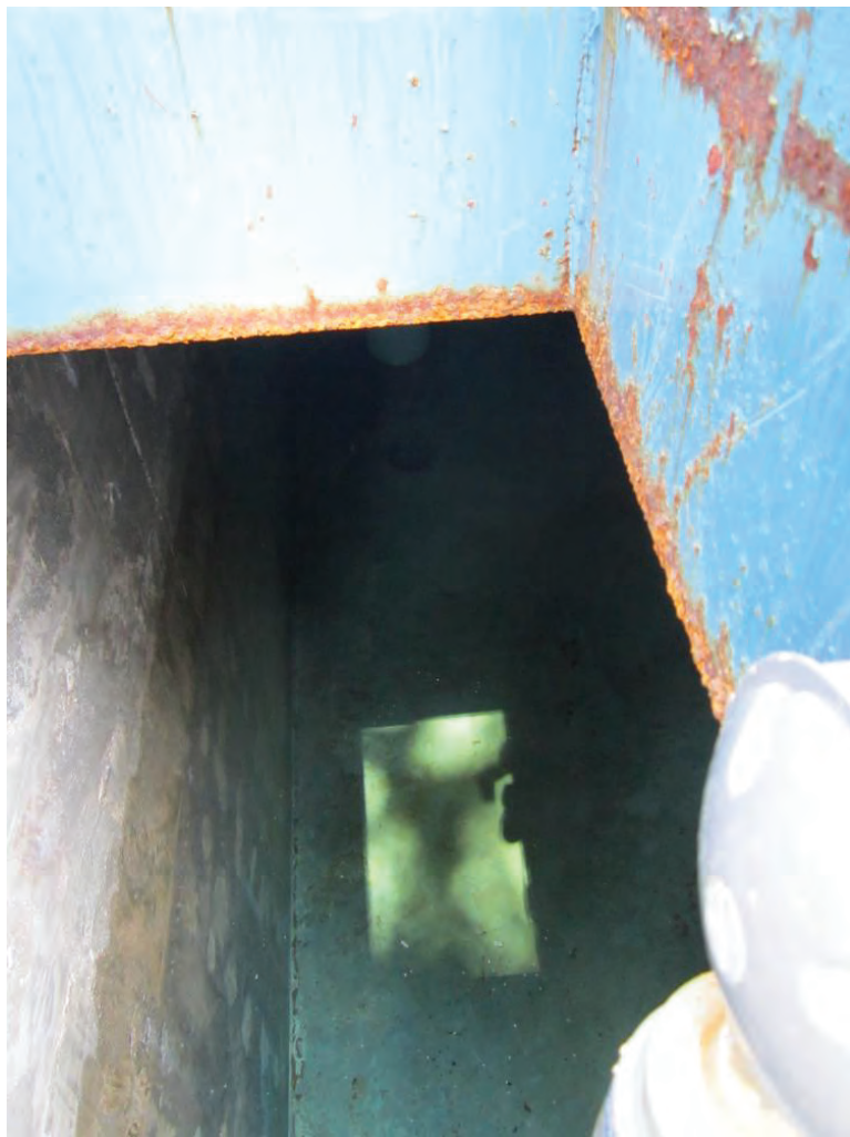
Photograph 82: Naples tank interior
