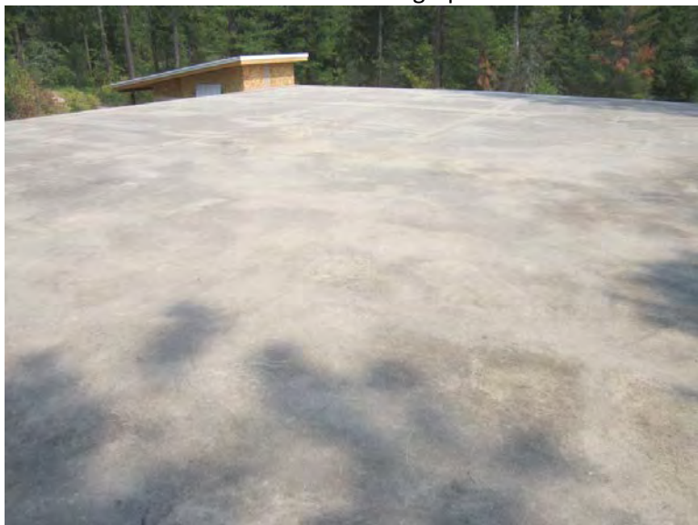
Photograph 81: Naples tank roof
