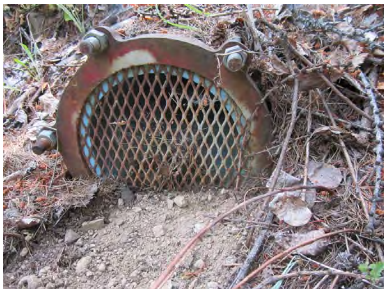
Photograph 68: Black Mountain reservoir screened drain
