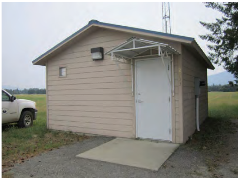
Photograph 47: Four Corners booster station
