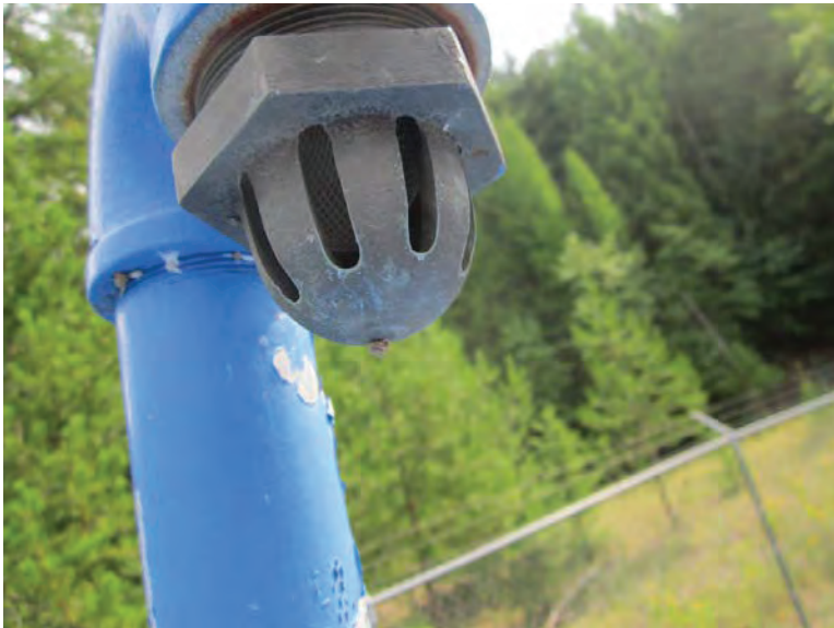
Photograph 55: Black Mountain reservoir vent w 24-mesh screen
