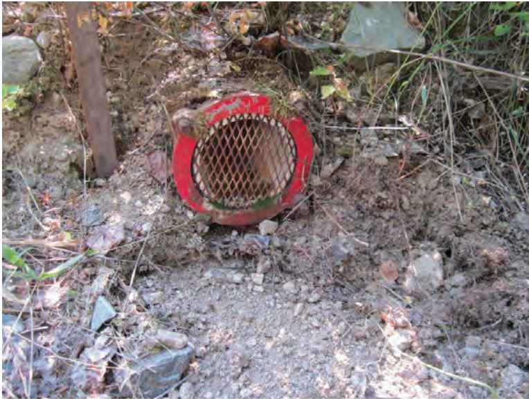
Photograph 69: Black Mountain reservoir screened overflow
