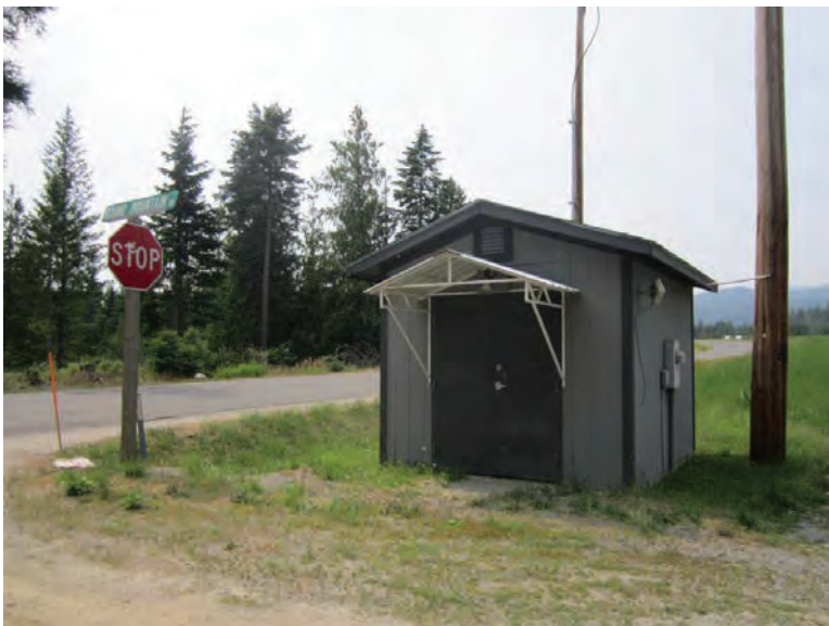
Photograph 99: Highland Flats booster station building
