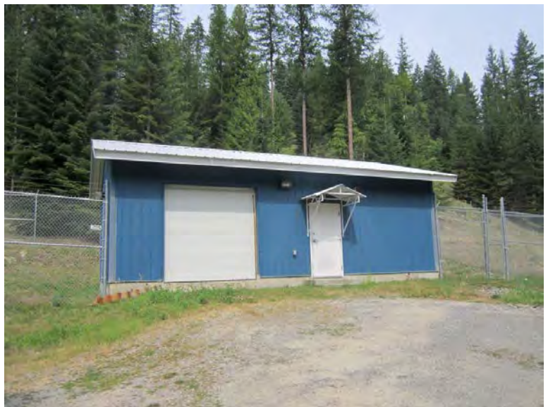
Photograph 24: Parker Canyon booster station
