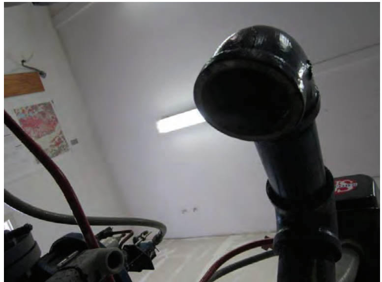
Photograph 4: Well 1 screened vent
