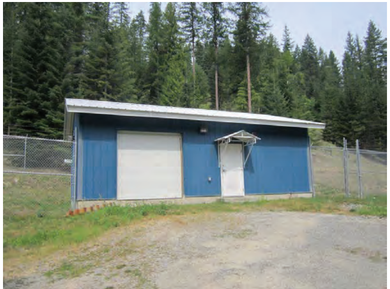
Photograph 24: Parker Canyon booster station
