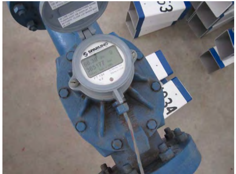
Photograph 44: Four Corners combined boosted flow meter
