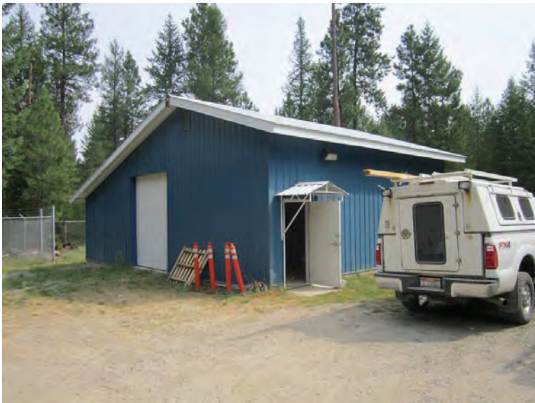
Photograph 23: Well 1 and 2 building
