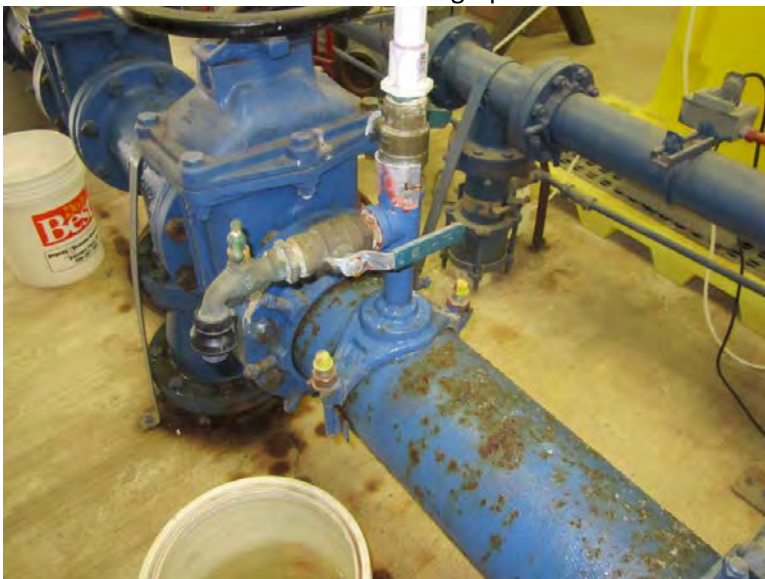
Photograph 17: Finished (chlorinated) sample tap
