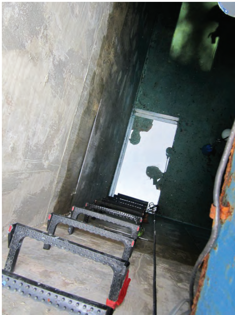
Photograph 84: Naples tank interior
