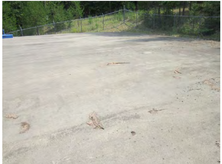
Photograph 56: Black Mountain reservoir lid
