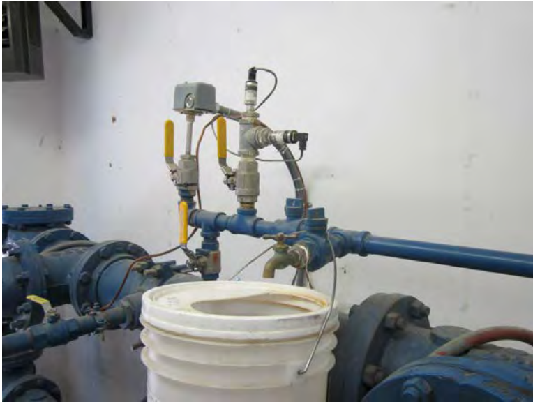
Photograph 97: Highland Flats pressure transducer and sample tap
