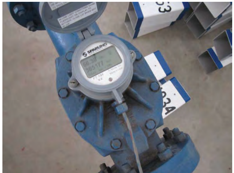
Photograph 44: Four Corners combined boosted flow meter
