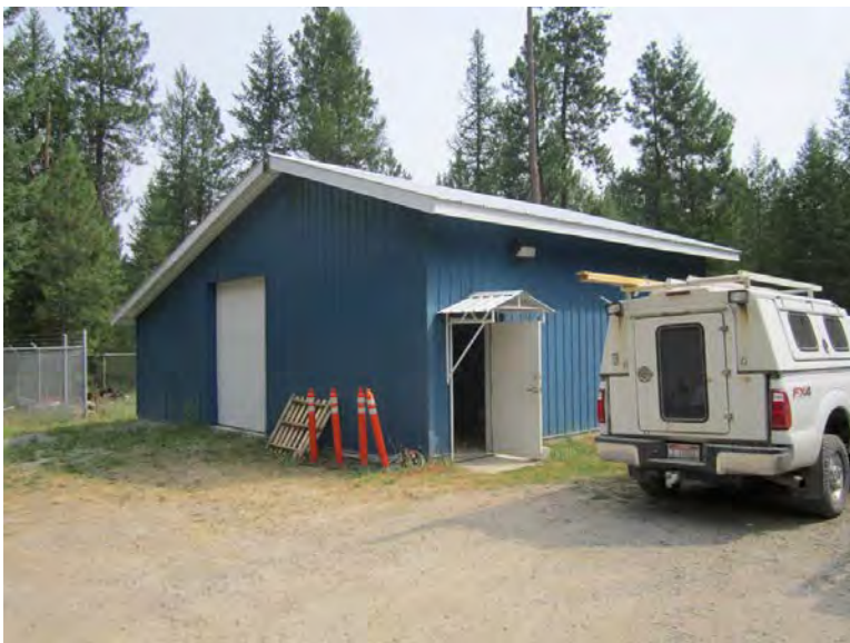
Photograph 23: Well 1 and 2 building
