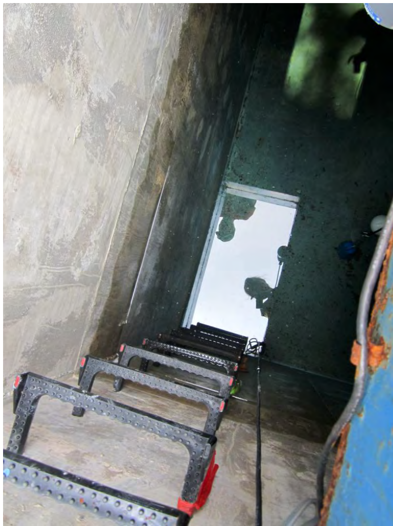
Photograph 84: Naples tank interior
