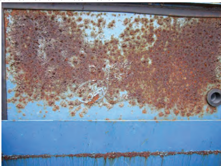
Photograph 86: Naples tank lid w water tight seal
