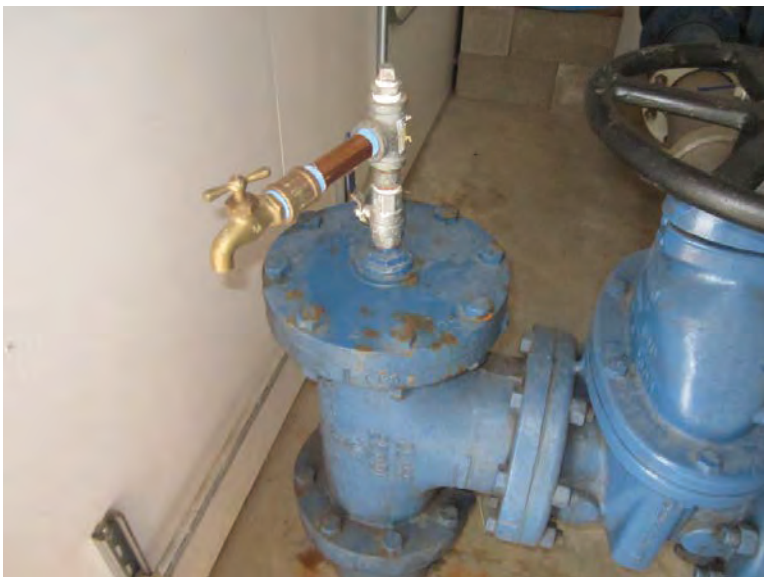
Photograph 43: Four Corners sample tap
