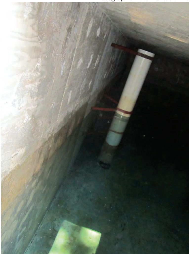
Photograph 85: Naples tank overflow
