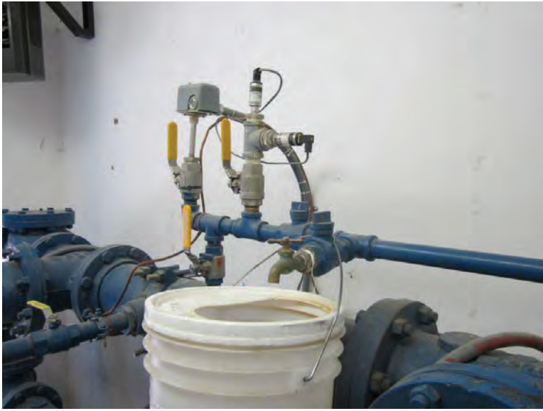
Photograph 97: Highland Flats pressure transducer and sample tap
