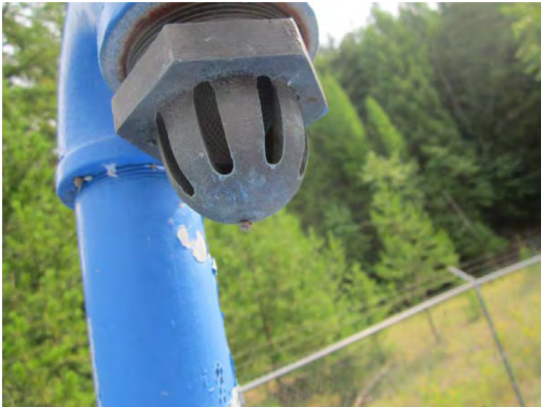
Photograph 55: Black Mountain reservoir vent w 24-mesh screen
