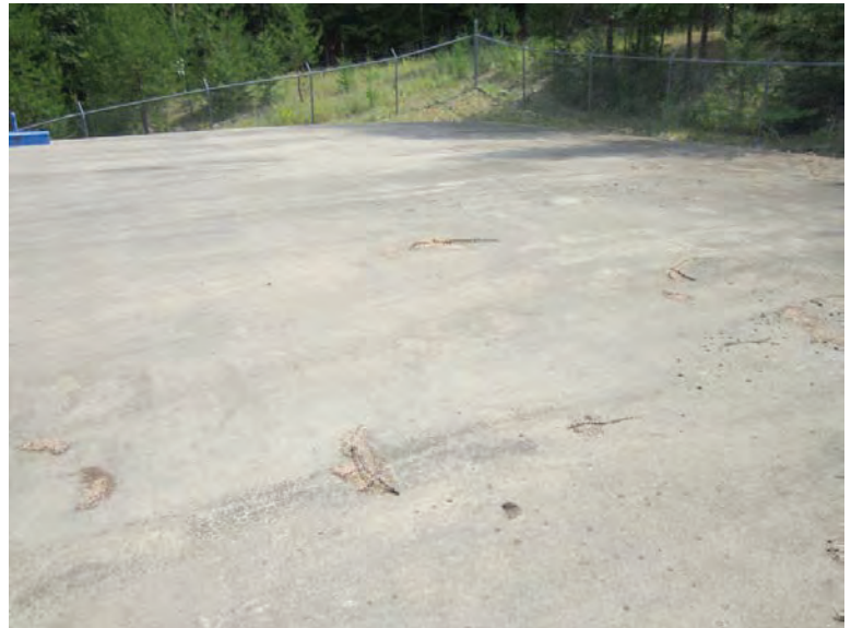
Photograph 56: Black Mountain reservoir lid
